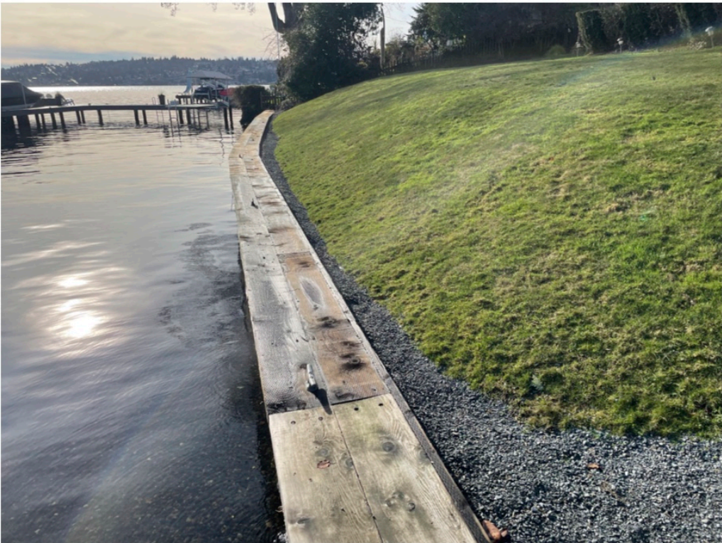
Photo 6 - Shoreline looking south along bulkhead.
